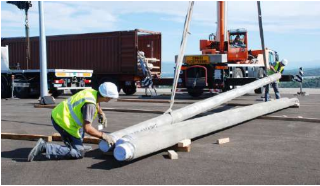
Figure B.2.5 First batch of piping delivered to ITER site, France
